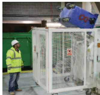
Waste containers are stored in the basement of the building. The waste contractor takes segregated materials for recycling and residual waste for further segregation.
