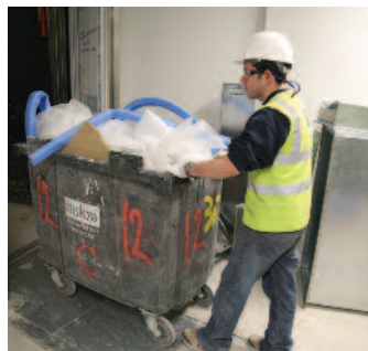
Waste materials are removed from occupiers' areas at the end of each day, providing a well organised working environment.
